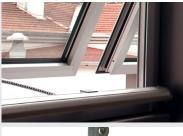
Tailored profile lengths according to the window frame width (International patent).
